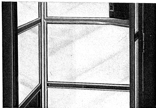
Fig. 10 – KS-16797, List 76 Shelf Installed
